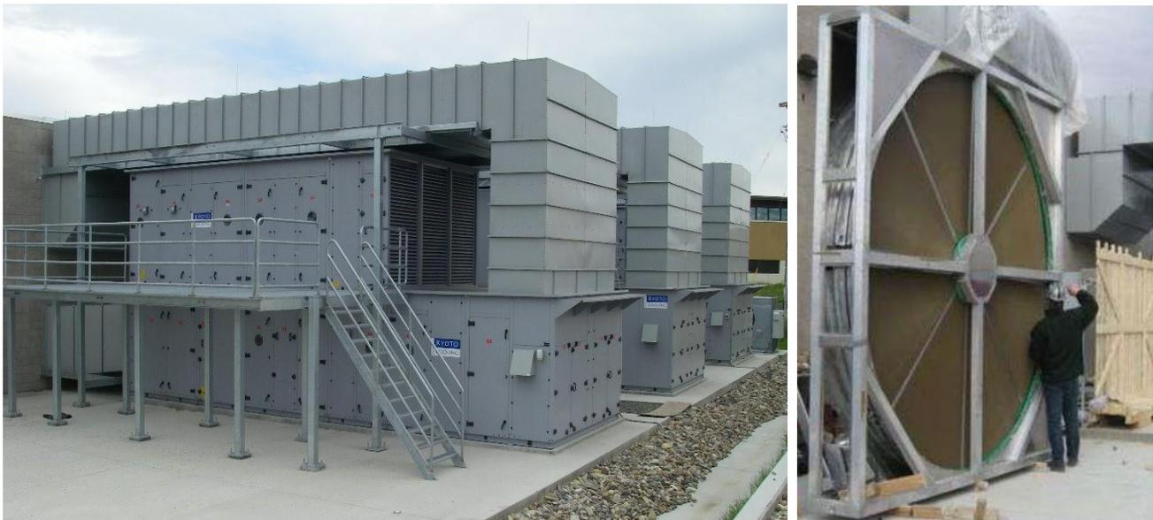
Air-to-air energy recovery wheel at Montana State Data Center. Photos courtesy of MTDEQ.
