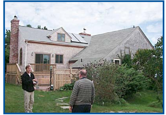
PV provides year round solar-assisted power to a domestic water-heating system for this residential addition in Rhode Island. Photo courtesy of NREL.
