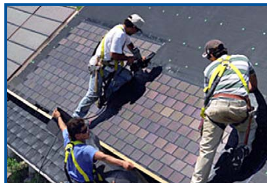
Photovoltaic (PV) shingles are an attractive solar option, since they look much like ordinary roofing shingles, but they also generate electricity. Photo courtesy of NREL.
