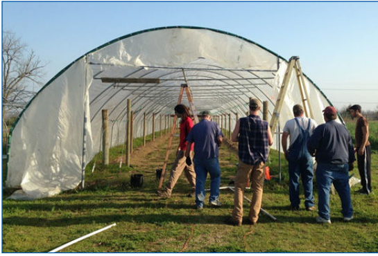
Putting the finishing touches on a high tunnel intended for table grapes at the University of Arkansas research farm. Note the grape trellis already in place. Building trellises is best done before the tunnel goes up. Photo: Susan Alman, University of Arkansas
