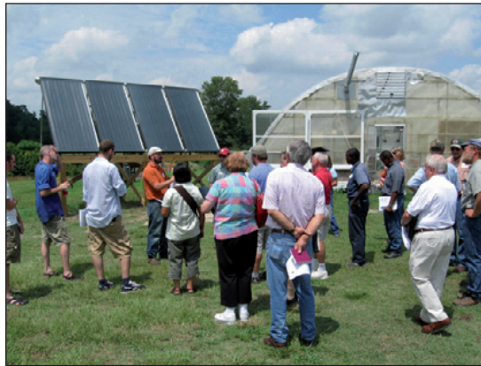
This solar water-heating system in North Carolina cost $8,000 to install and saves $2,000 per year in propane costs for space heating. Photo: Mike Morris, NCAT
