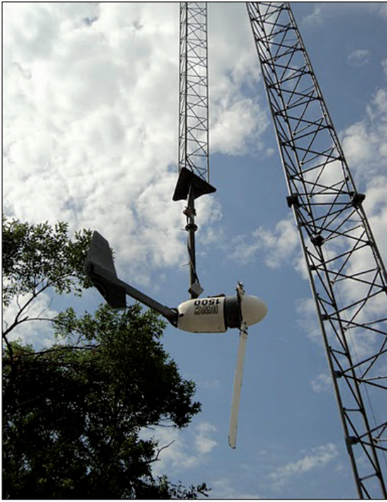
Winds reaching 100 miles per hour folded this tower in Iowa in half, causing the turbine to strike the tower. Photo: Rich Dana, NCAT
