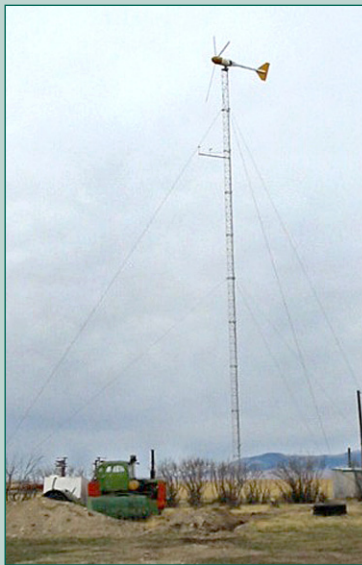
Guyed-lattice tower. Photo: Windustry.org
