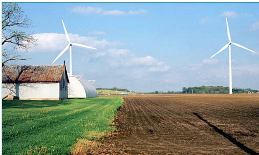
Wind turbines operate in harmony with farming and ranching. Photo: NREL/PIX14070
