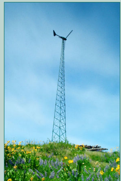
Lattice tower. Photo: Windustry.org
