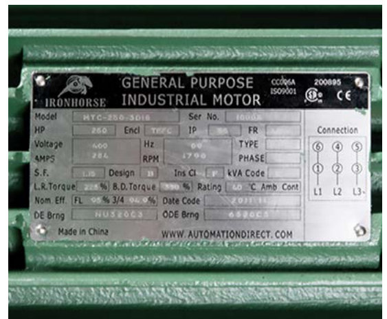
Figure 4. Nameplate of a 250-horsepower motor. Photo: NCAT
