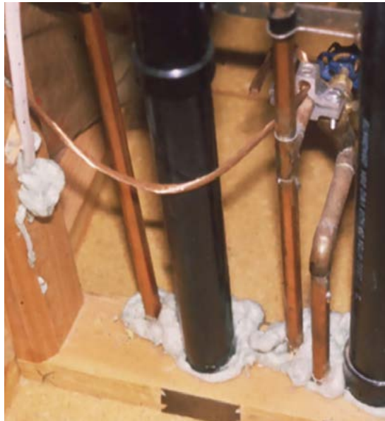
Figure 6. Well-sealed air leaks around plumbing. Photo: NCAT
