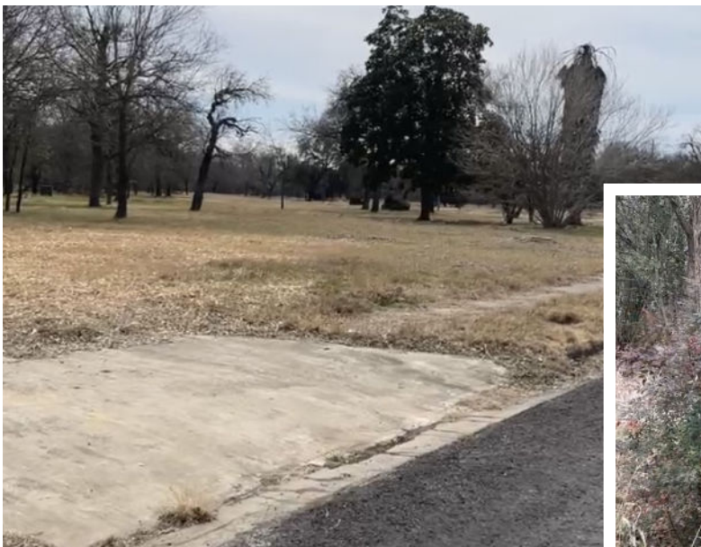
Driveway aprons in need of removal after a buyout demolition in the Upper Onion Creek floodplain.
