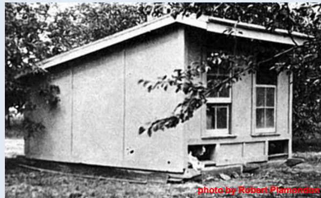
Traditional all-season colony house used in the past. For extra ventilation in summer, the window sashes are removed and a full-width vent in back is opened under the eaves.
