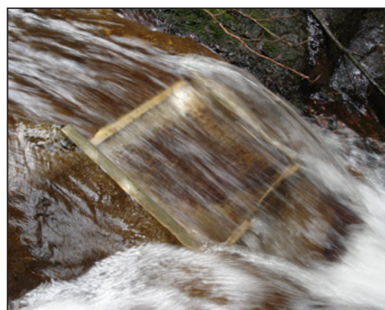
An intake can be integrated into the stream bed to capture only a small part of the flow and minimize environmental impacts. Photo: Leif Kindberg, NCAT
