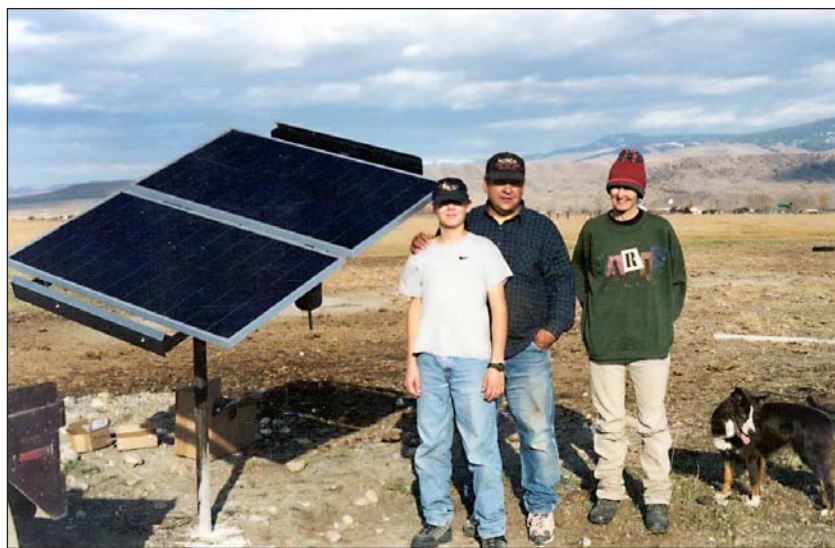
This solar pumping system on the Hirsch Ranch near Deer Lodge, Montana, is protecting stream banks along Racetrack Creek, an important trout spawning stream. Photo: NCAT
