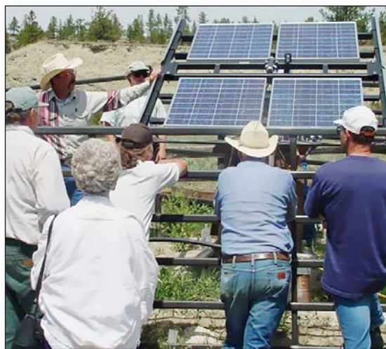
A tracking PV array replaced an old and unreliable windmill on the Ballard Ranch near Lavina, Montana. Photo: NCAT
