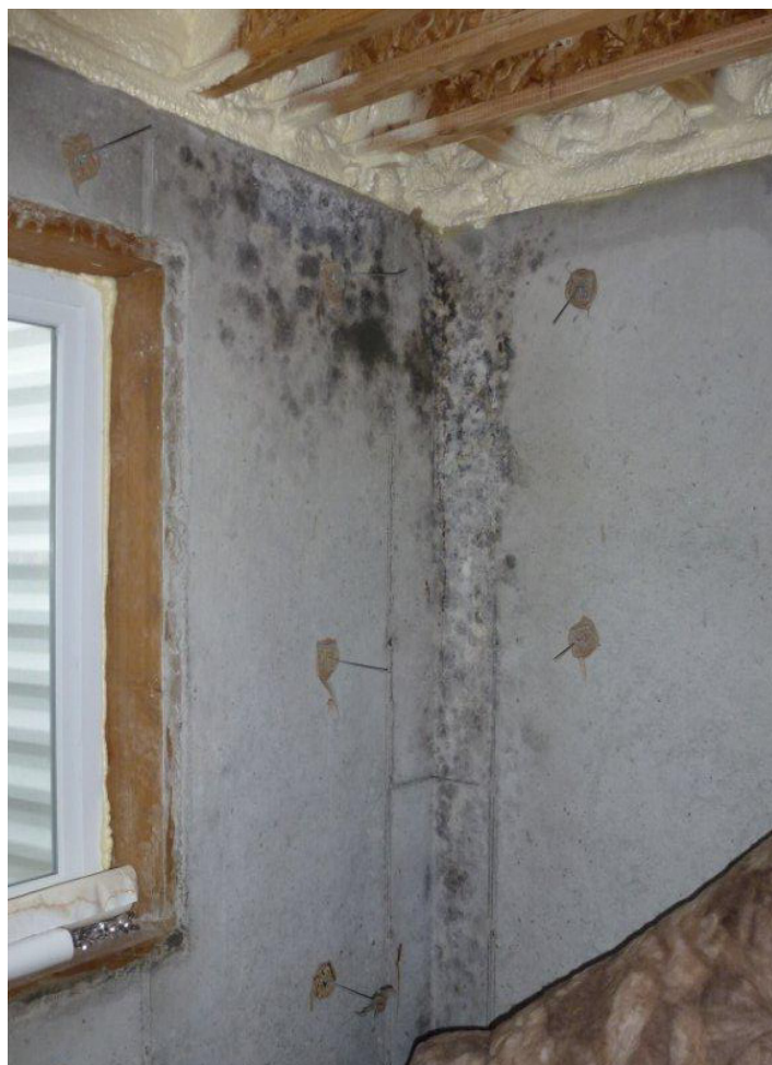
Figure 8-4. Inadequate Mechanical Ventilation Can Contribute to Mold and Other Moisture-Related Problems
