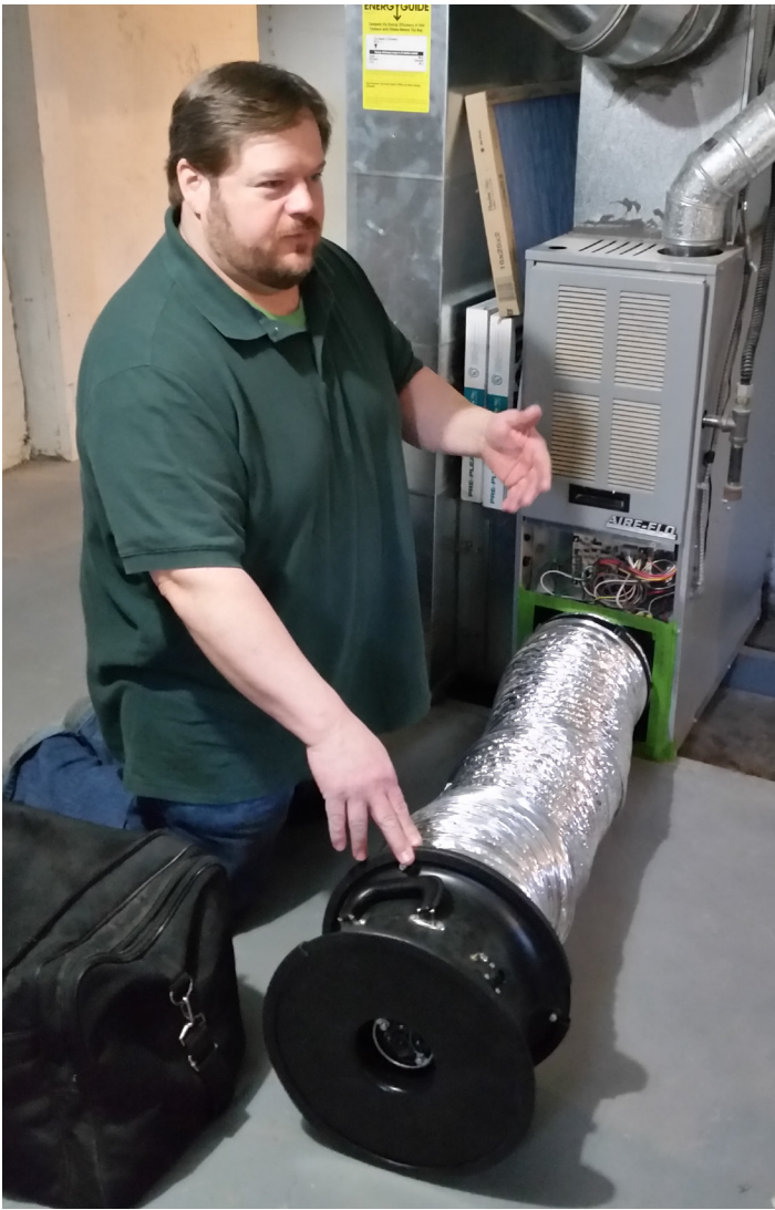
Figure 7-13. Duct Tester Fan Mounted at Base of Air Handler Cabinet
