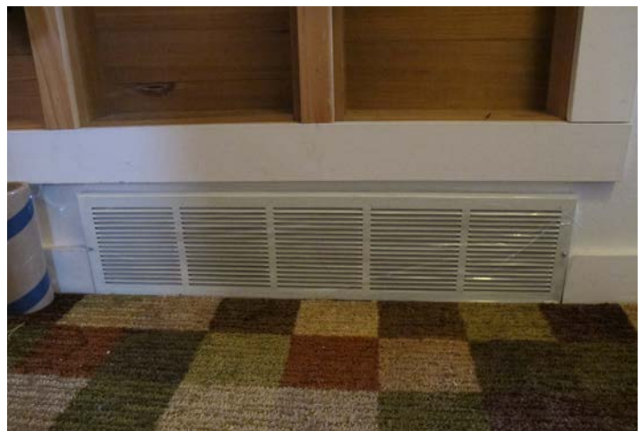
Figure 7-5. Sealing Registers Testing occupied homes can make locating all registers a real challenge.
