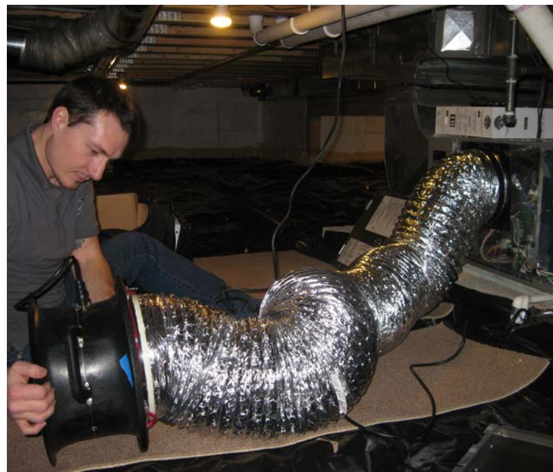
Figure 7-11. Duct Tester Fan Mounted at Crawlspace Heat Pump
