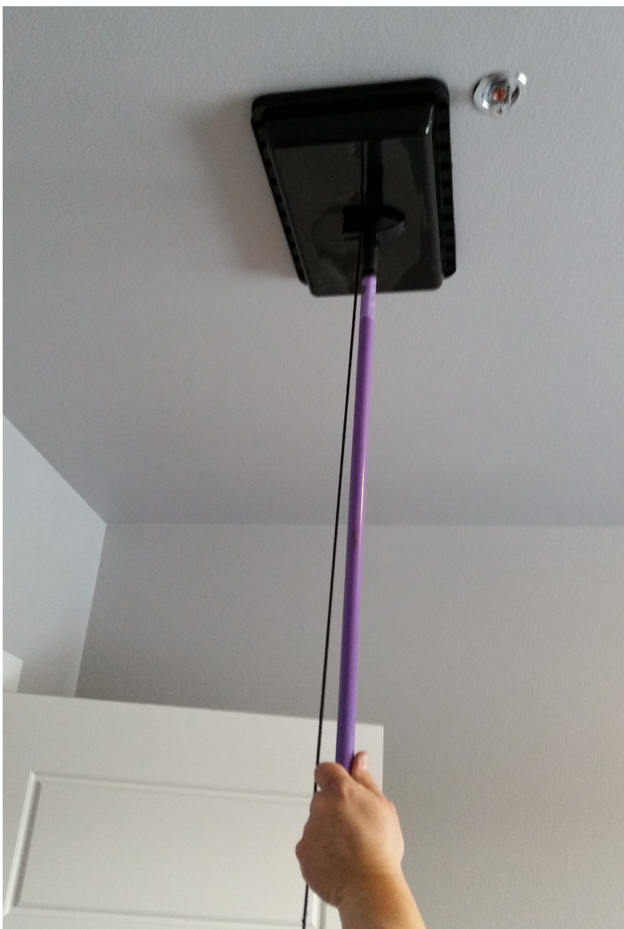
Figure 7-3. Sealing Registers
