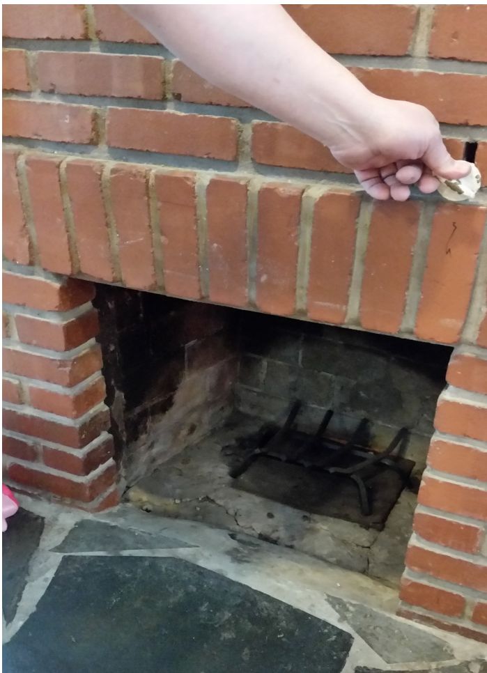
Figure 6-11. Close Chimney Dampers and Combustion-Air Inlets on Solid Fuel Appliances
