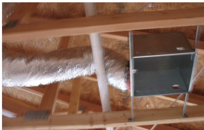
Figure 8-3. Long or Crimped Exhaust Fan Ducts Reduce Actual Exhaust Airflow
