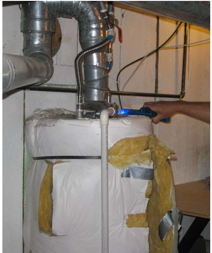
Figure 10-4. Flue Spillage Test
