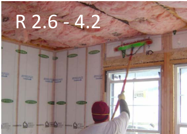
Batt Insulation In Ceiling
